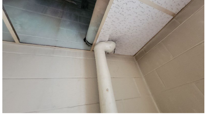
Photo 2 (April 7, 2023): PACM pipe insulation and fitting identified in the janitor's closet on the first floor of the 1968 addition.
