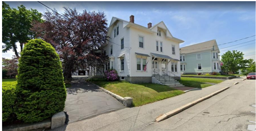
Figure Cb4: View of residential context from Birch Street
