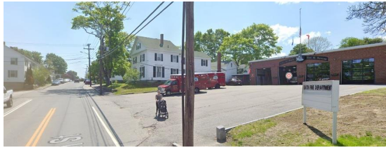
Figure Ca2: View of existing central station from High Street
