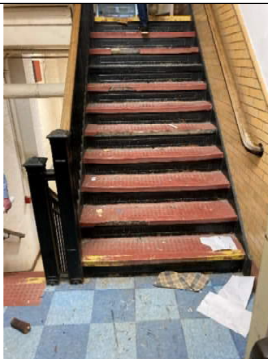
Existing 1928 egress stair.
