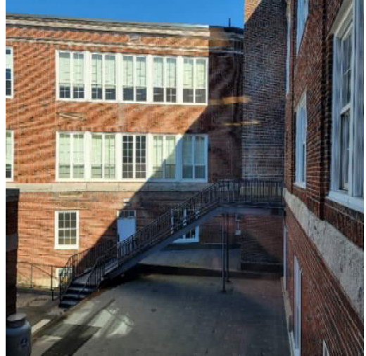
New Fire Escape Stair from Auditorium.
