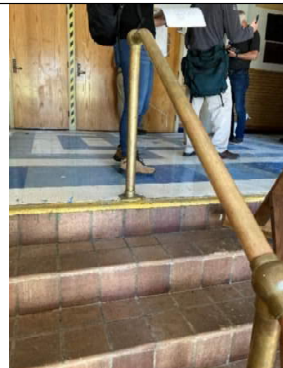
Existing 1928 main entry stair.
