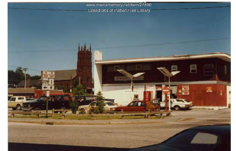
Fig. 7: Vine & Water Street intersection in 1986, former site of the Bath Opera House Source: Patten Free Library/Maine Memory Network
