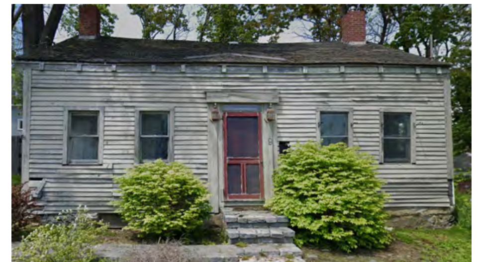
Fig. 13: 9 Fremont Street, to be demolished Source: Bath Code Enforcement Office
