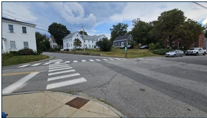
The Concept Plans start at the intersection of Commercial Street/Front Street/Oak Street. The study proposes to convert the intersection into an all-way stop and provide geometric improvements (especially to the southwest corner) that would reduce the overall size of the intersection, thereby shortening crosswalks and improving pedestrian desire lines. The plans show an additional pedestrian landing at the
