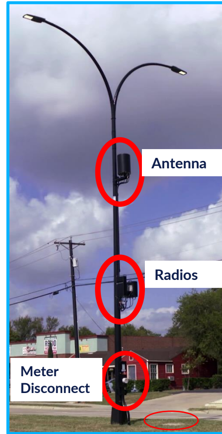
Power/fiber handhole
